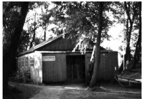
Club house No. 3 South Dinghy park 1970.
