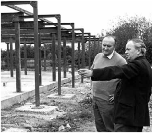
Foundations are laid. John Jones and Sir Frank Cooper.
