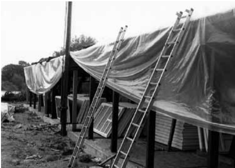
Current clubhouse, without panels or second floor.
