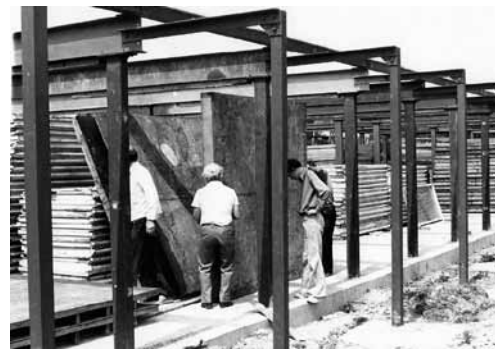
Current clubhouse steel frame and panels.
