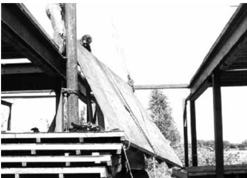
Block and tackle used in the construction.
